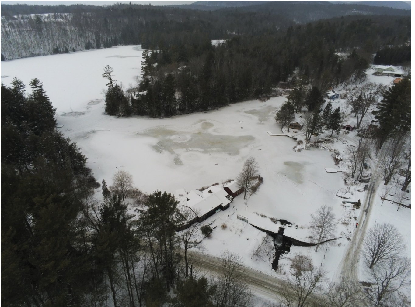
Figure 10 Curtis Pond Dam in Calais
