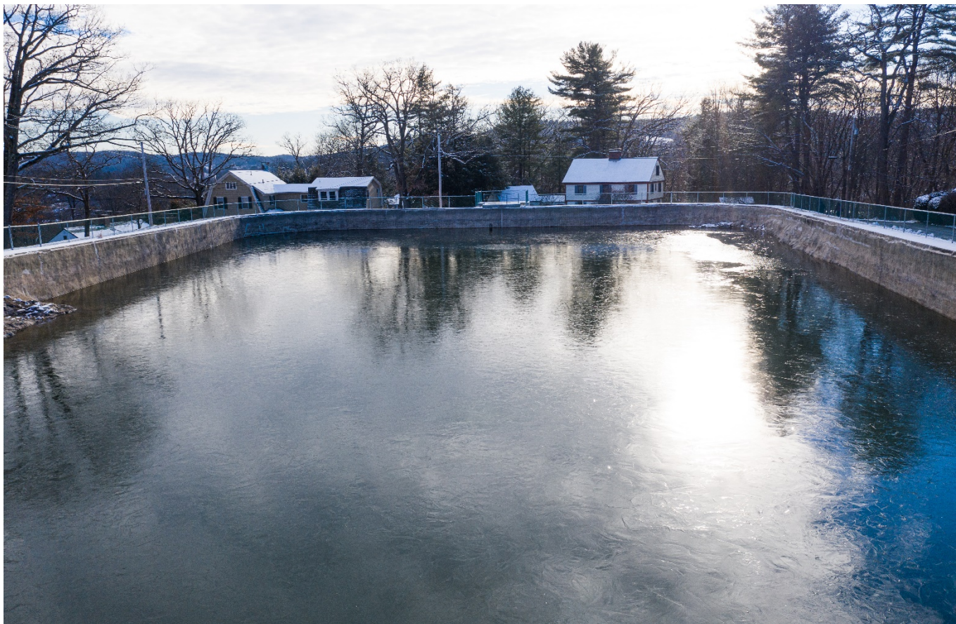
Figure 12: Chestnut Hill Reservoir Dam in Brattleboro
