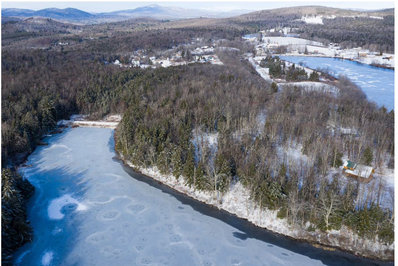
Figure 15: Lake Sadawga West Dike in Whitingham
