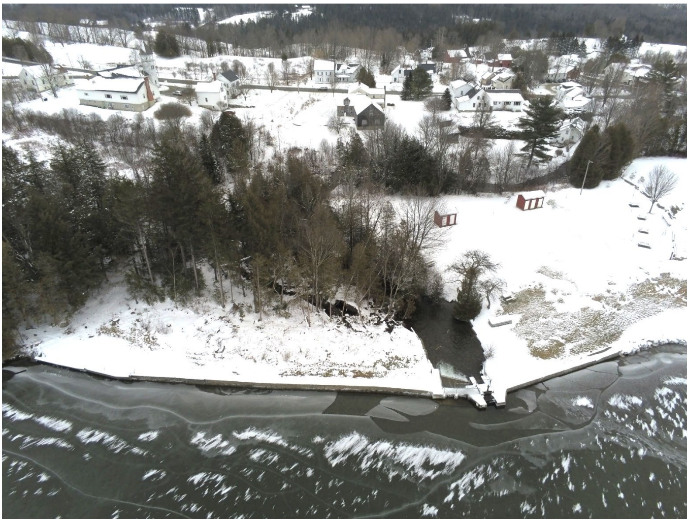
Figure 17: Caspian Lake Dam in Greensboro
