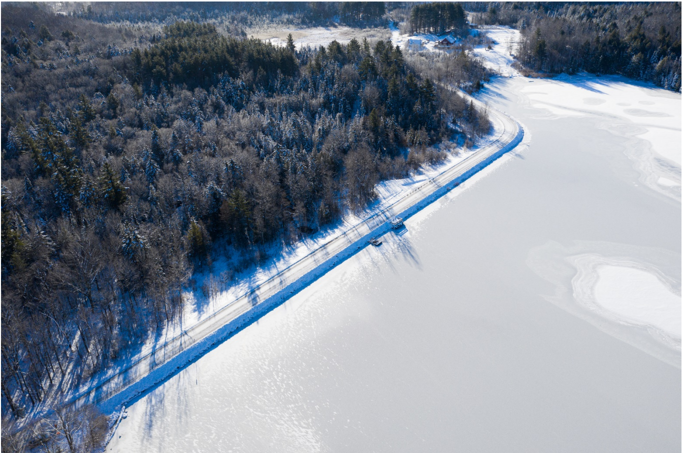
Figure 18: Kent Pond Dam in Killington
