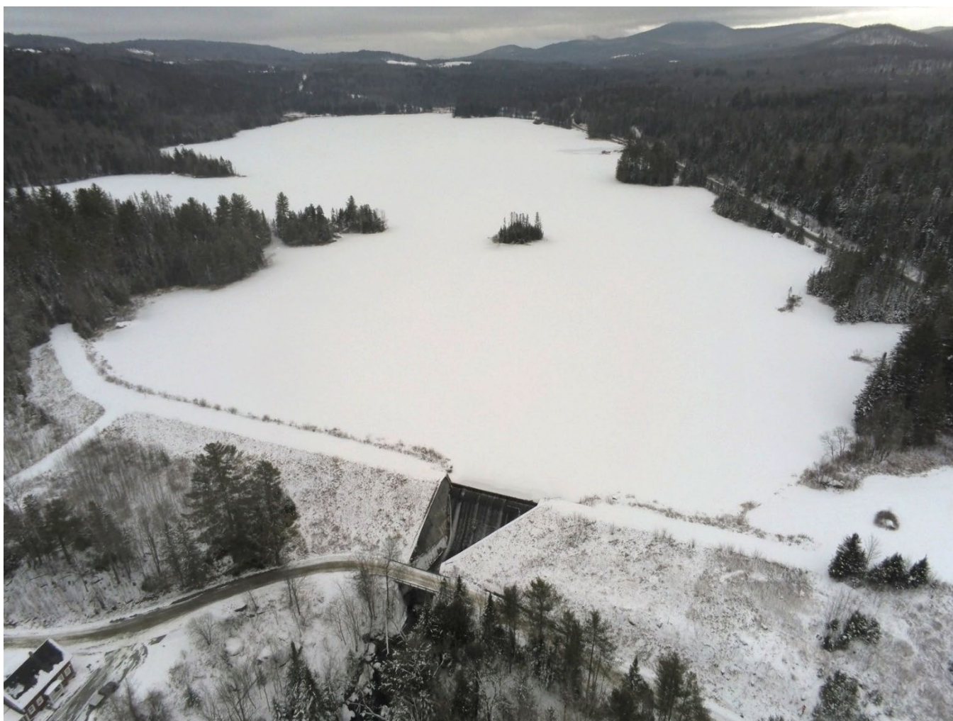
Figure 16: Thurman W. Dix Reservoir Dam in Orange
