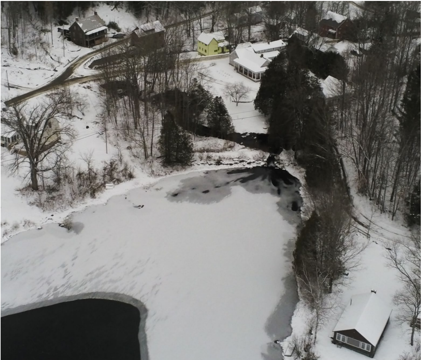
Figure 13: Mirror Lake Dam in Calais
