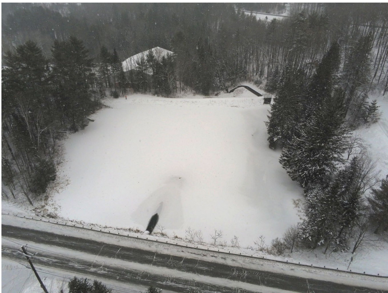
Figure 11: Institute Pond Dam in Lyndon
